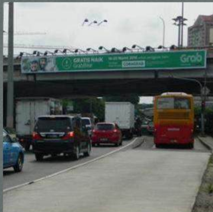
UNDERPASS AHMAD YANI JAKARTA PUSAT
